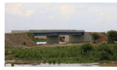
The view of the Sibiti Bridge after its completion, it has a span of 82 meters.
